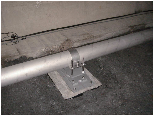
Fig. 4.2.24. Support for the vacuum duct.
