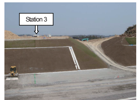
Fig.2.4.2. Array observation site of station 3. This photo was taken from station 5.
