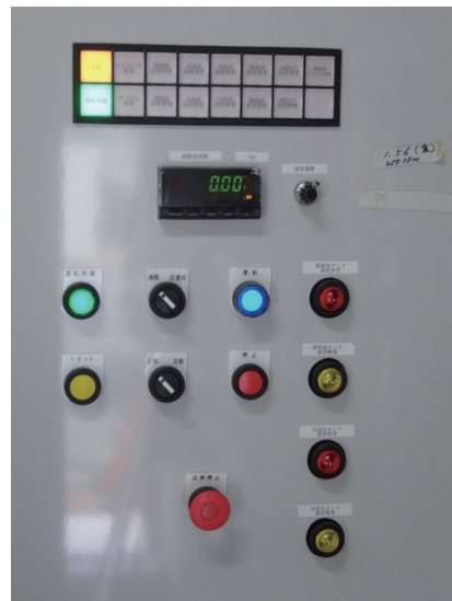
Fig. 2.2.7. Alarm panel of the ACROSS transmitter. When the status parameter (e.g., coolant temperature) exceeds (or falls below) the critical value, the corresponding light turns on.
