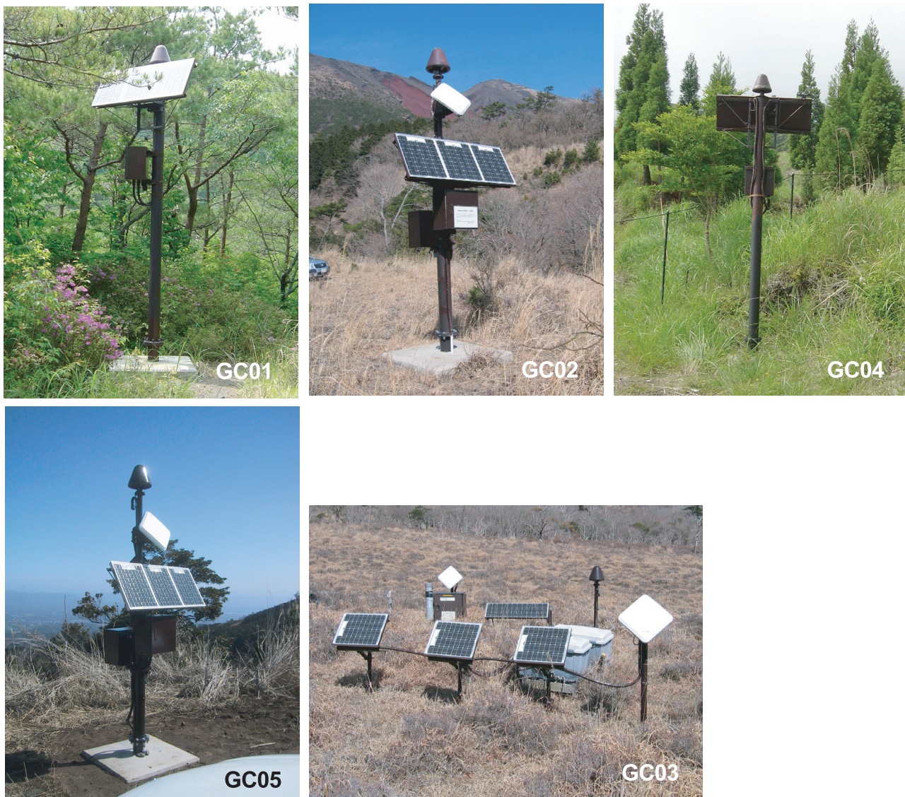
Photo 2.1.2.1 Continuous GPS observation site on Kirishima volcano installed by MRI.
